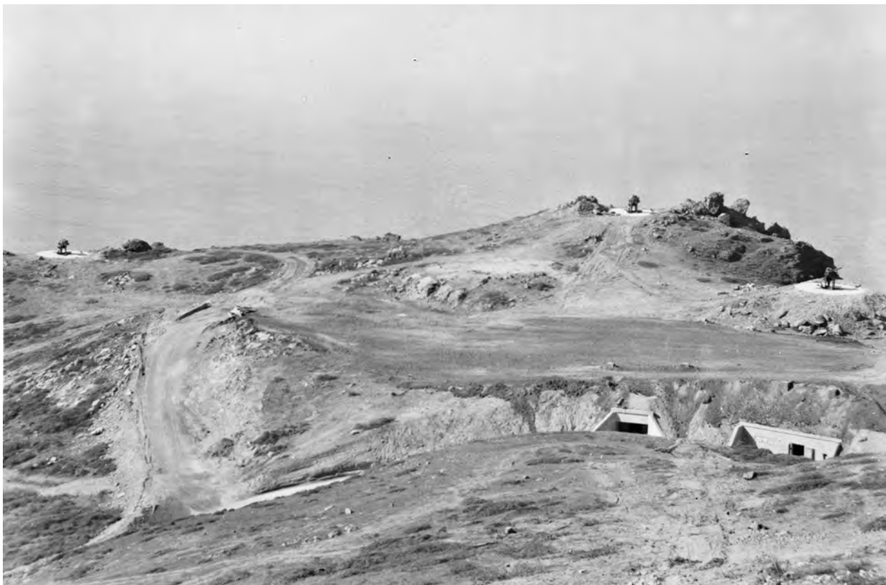
3. AA Battery No. 1 and supporting structures. GGNRA Park Archives, GOGA-2316.
