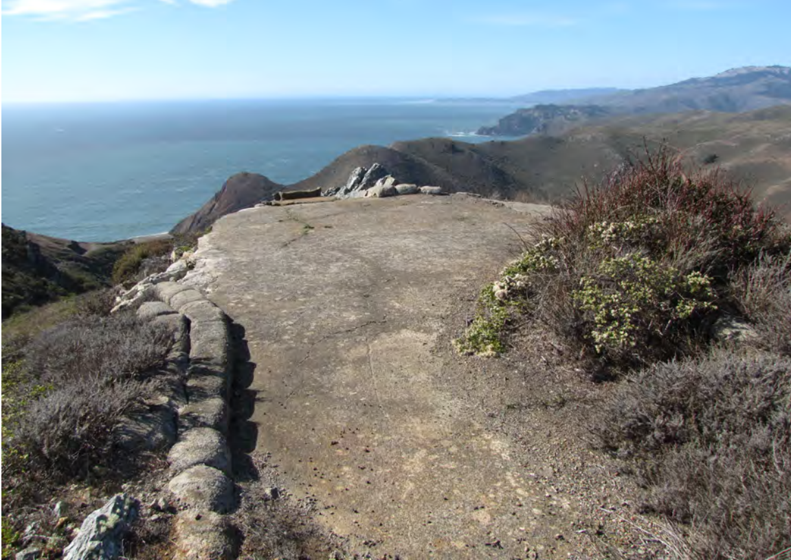
12. Concrete pad that may have been used for a generator. Photograph by author, October 21, 2014.
