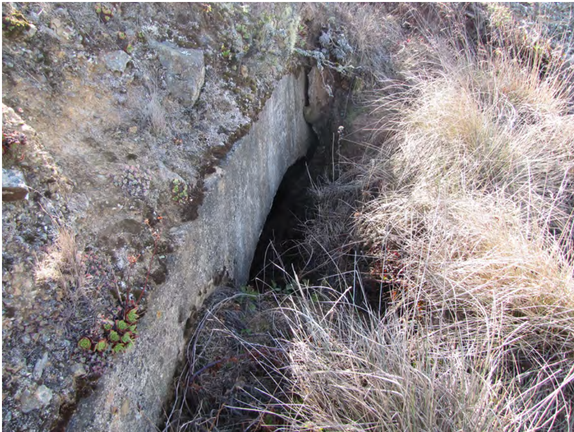
15. Semi-buried entrance to underground hutment with concrete roof, below Gun Block No. 1.
