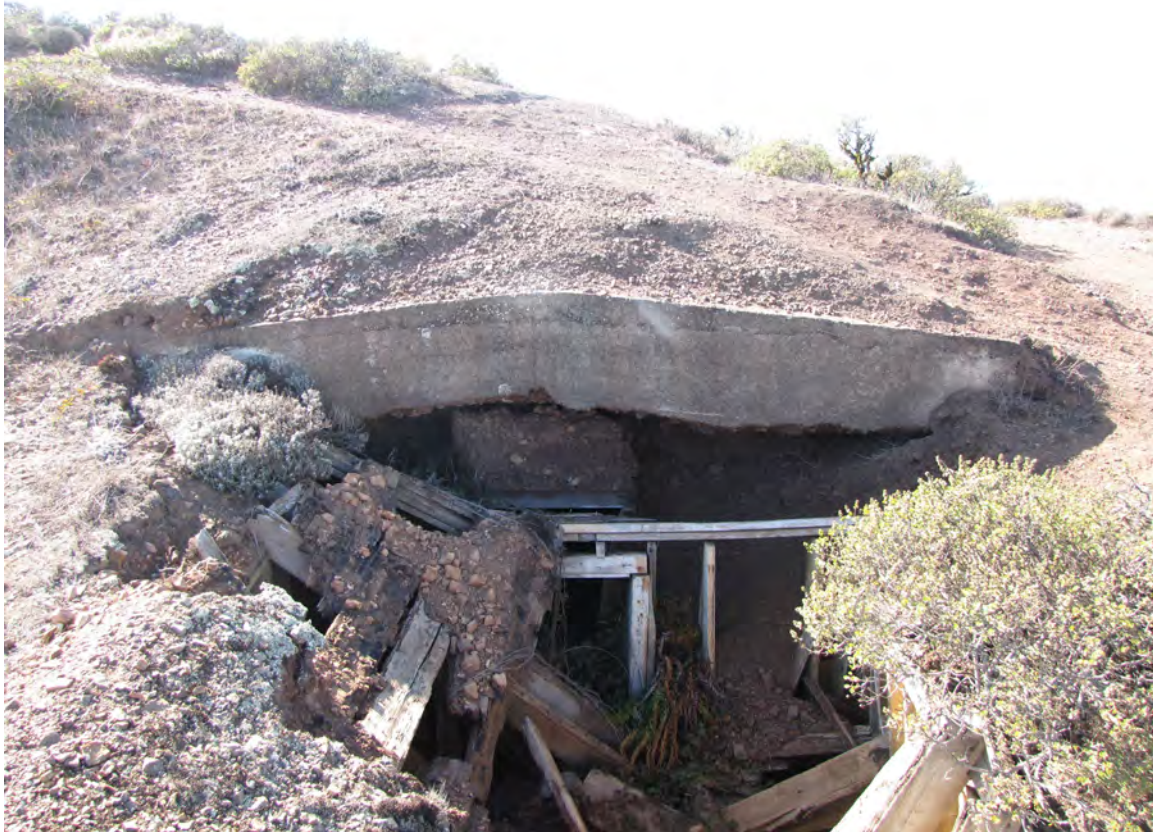
10. Collapsed anteroom entrance to underground corrugated steel shelter with 2-foot-thick concrete roof below height-finder pit. Photograph by author, October 21, 2014.
