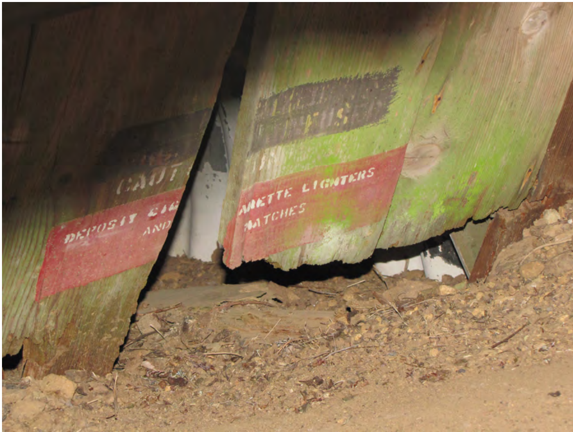
16. Surviving painted stencil inside underground shelter below AA Gun Block No.1
