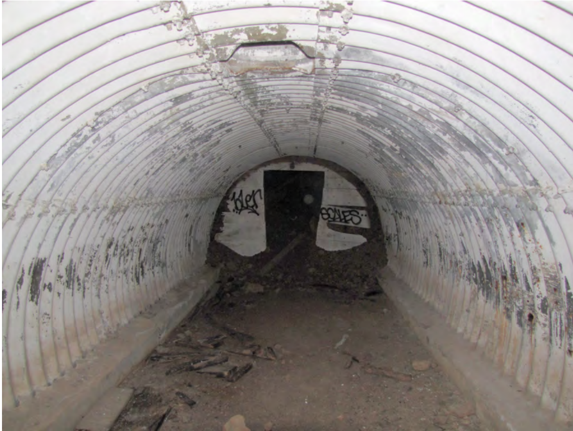
17. Interior of underground corrugated-steel shelter below AA Gun Block No. 2, October 21, 2014.
