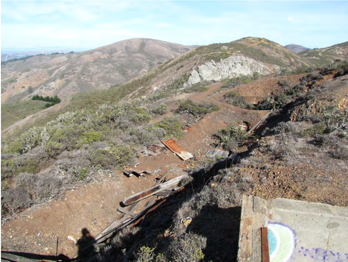
11. Collapsed day room/mess hall next to director pit. Photograph by author, October 21, 2014.
