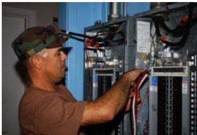
Figure 10. An electrician by day and citizen-soldier by night, Spc. Carlos Villasenor uses his civilian skills to good use. The San Diego resident took the lead and led contractors in powering up a school building that housed the 2/185 th Armor Battalion, California Army National Guard. The building was occupied by more than 200 Guardsmen, is the only structure with electricity in an 18-block radius in Orleans Parish. (69 th Press Camp Headquarters)
