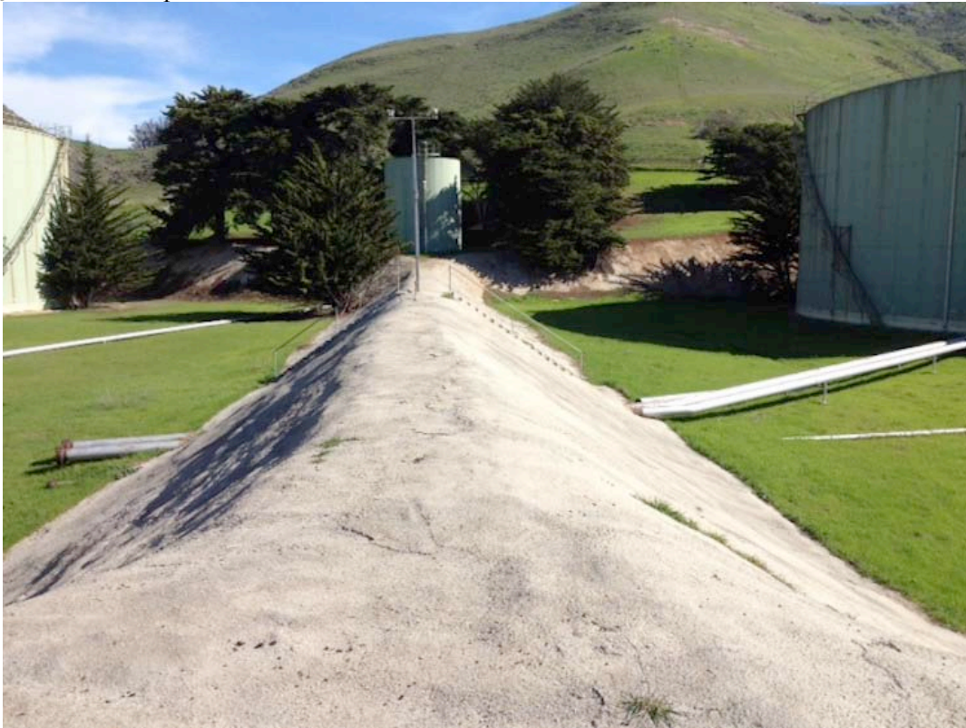
Water tank showing concrete berm. Facing east.
