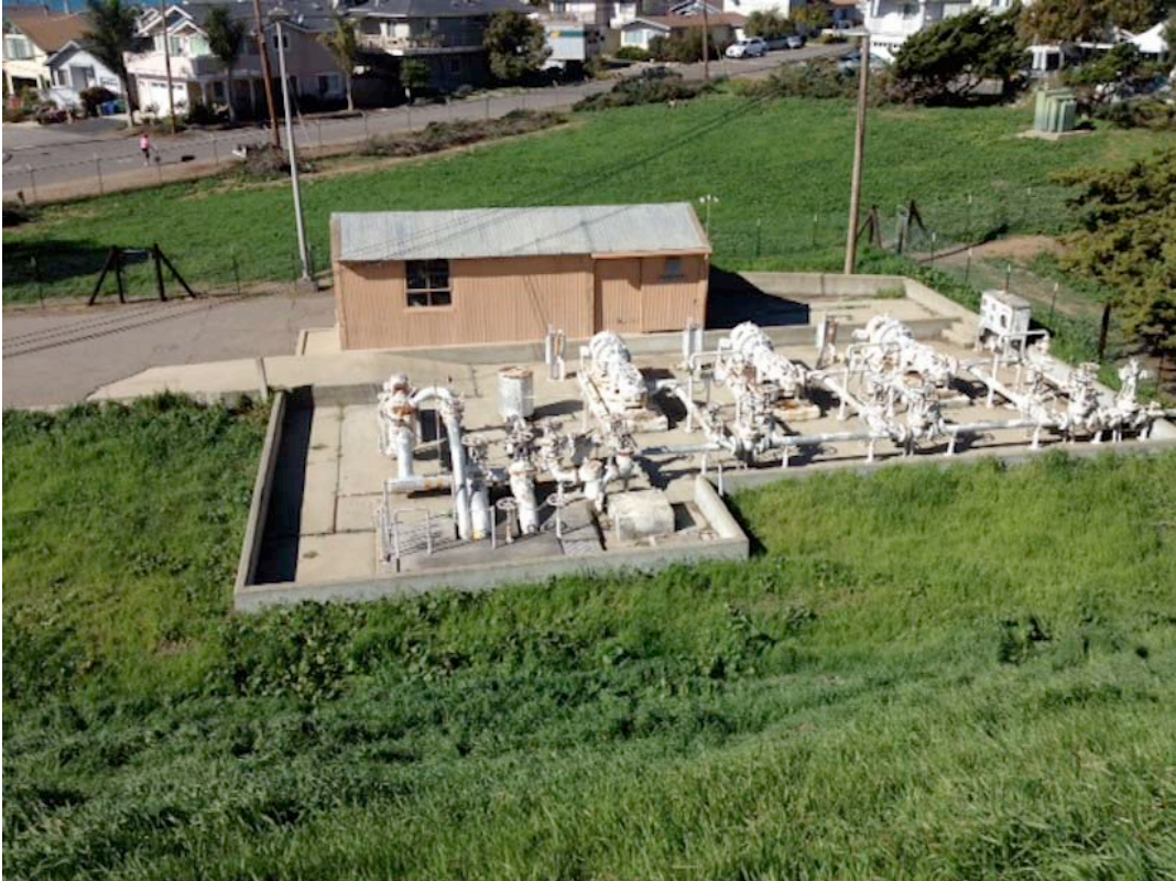
Pump house, showing fuel piping area. Facing northwest. Panorama Drive in left background.
