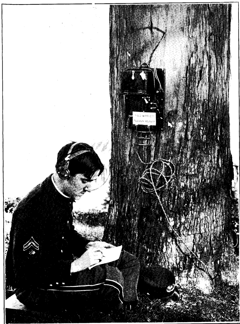
RECEIVING WIRELESS MESSAGES AT FORT MASON, CALIFORNIA, FROM YERBA BUENA NAVAL STATION, 3\frac{1}{4} MILES DISTANT. EUCALYPTUS TREE AS ANTENNA.
