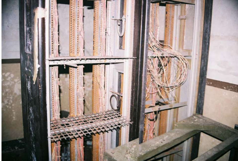
Surviving switchboards with the remaining wire lines and terminal boards inside the switchboard room. Matthew Kent
