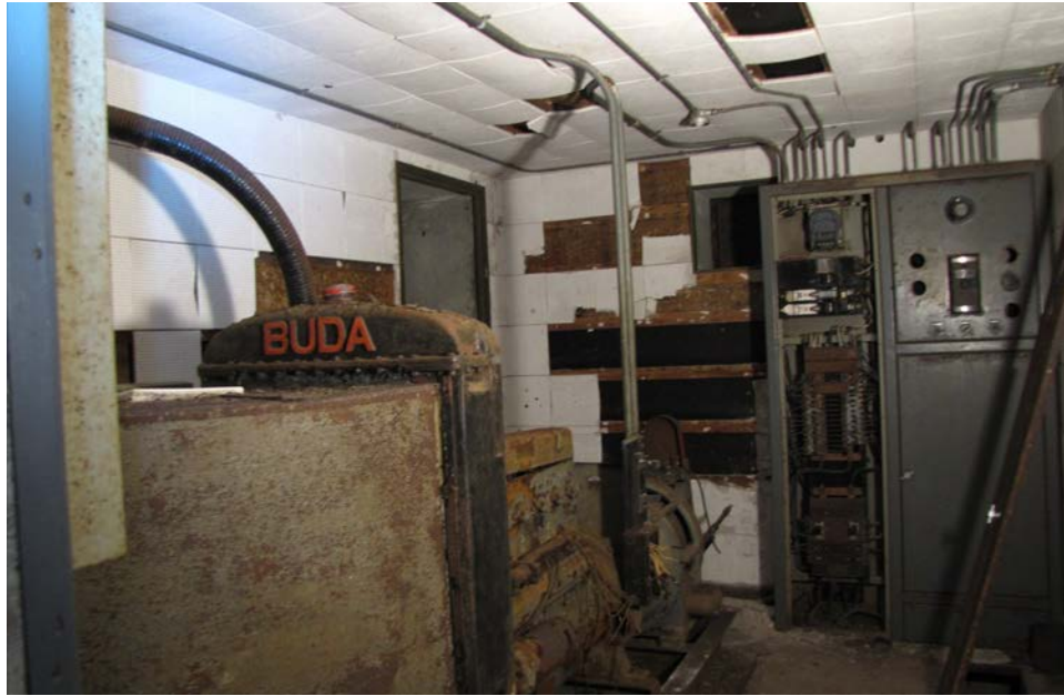
Largely intact power room inside the radio & switchboard room. Matthew Kent
