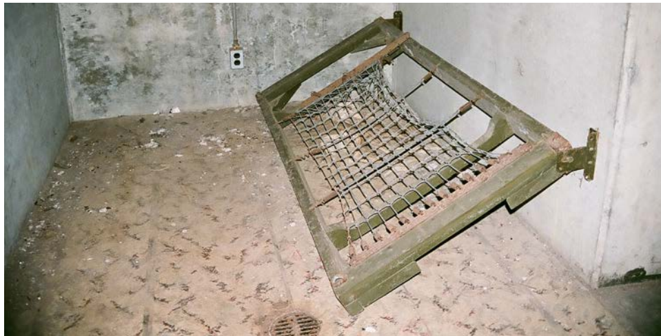
Prison-type metal bunk in the main corridor of the radio & switchboard room. Matthew Kent
