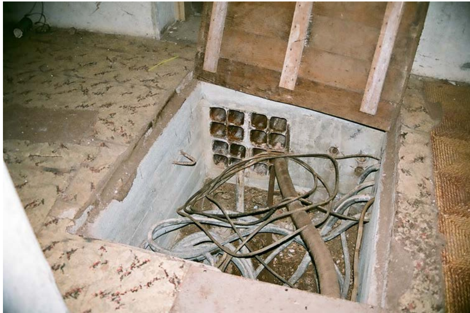
Cable manhole with intact cables, inside the main corridor of the facility. Matthew Kent
