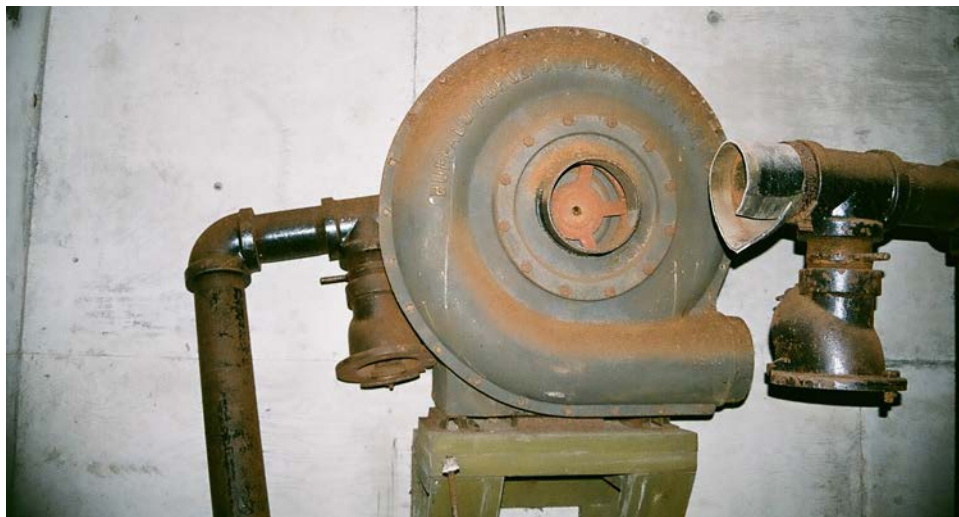
Buffalo Forge Co. blower unit inside the CWS (gas-proofing) room. Matthew Kent
