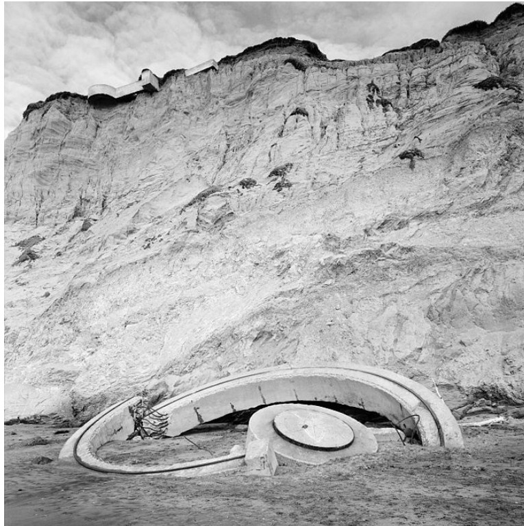
9. Collapsed Panama mount on beach as seen in Figure 8. Exposed underside to extant Panama mount and ammunition depot are seen at top of cliff left of center. Looking 342° NNW. - Fort Funston, Panama Mounts for 155mm Guns, Skyline Boulevard & Great Highway, San Francisco, San Francisco County, CA. HAER CAL,38-SANFRA, 214A—6. http://hdl.loc.gov/loc.pnp/hhh.ca2388/photos.190949p
