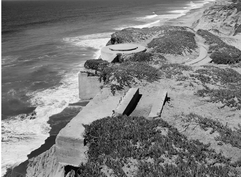
8. Panama mount in rear. Foundation in foreground is base for ammunition depot. Looking 328° NNW - Fort Funston, Panama mounts for 155 mm Guns, Skyline Boulevard & Great Highway, San Francisco, San Francisco County, CA. HAER CAL,38-SANFRA, 214A—3. http://hdl.loc.gov/loc.pnp/hhh.ca2388/photos.190946p
