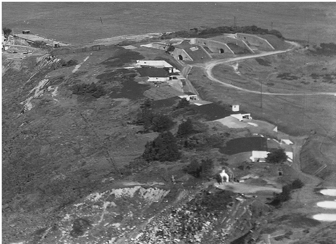
Fig. 27. The “new” incinerator at the dump site, lower right, February 1935. Courtesy GG Bridge, Hwy & Trans. Dist.
