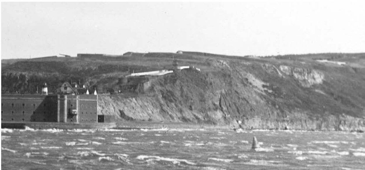
Fig. 33. The terraced superior slopes of Endicott-era batteries are visible above Fort Point in this c. 1900 view. A 12-inch disappearing rifle at Battery Lancaster appears at left. Courtesy California Historical Society.
