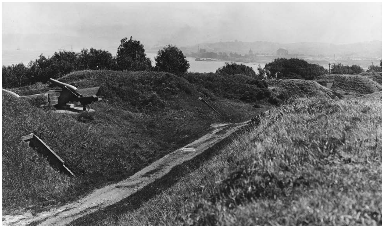
Fig. 17. A pair of 8-inch rifled Rodmans and the covered way behind East Battery, 1915. The Panama Pacific International Exposition can be seen in the distance. GOGA, FOPO Collection.
