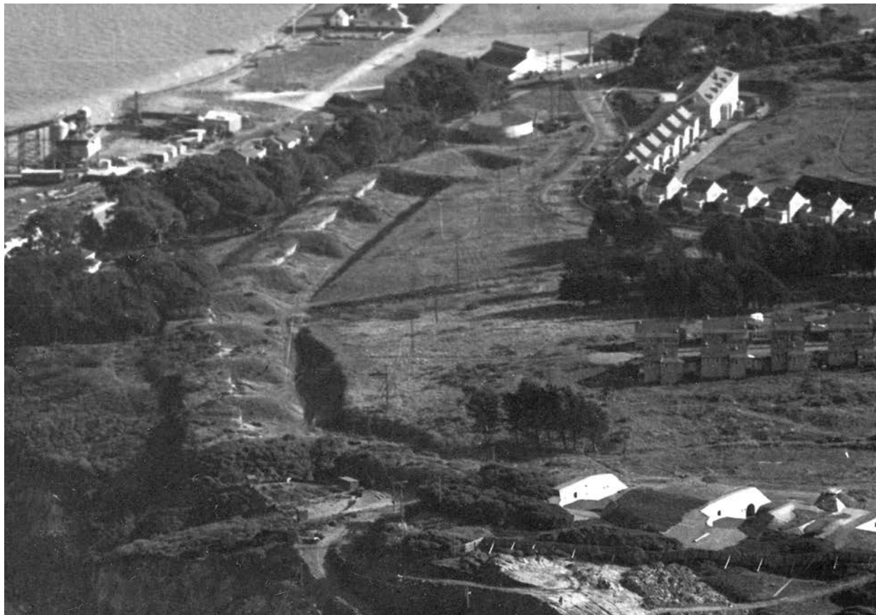
Fig. 13. Aerial view of East Battery in 1934, before construction of the Golden Gate Bridge toll plaza, showing the covered way and parados behind the emplacements. Battery Lancaster is at lower right.
