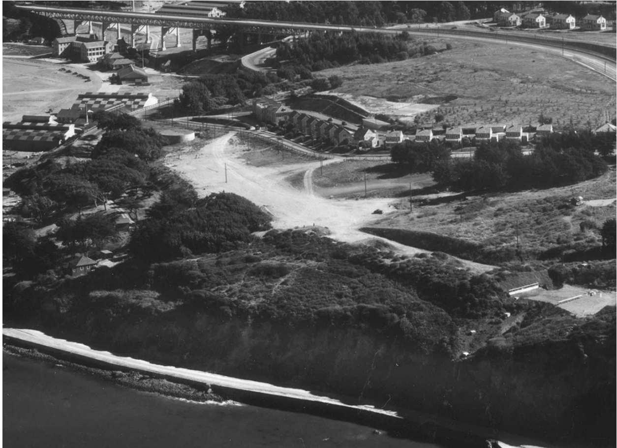
Fig. 34. East Battery partially filled, October 1937. Compare to 1934 conditions in Fig. 13. Courtesy GG Bridge, Hwy & Trans. Dist.
