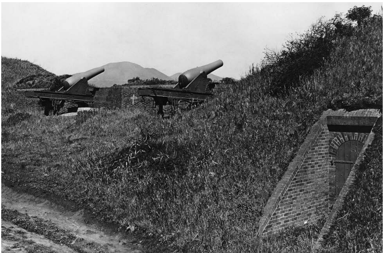
Fig. 5. A “Plan of 1870” two-gun emplacement at East Battery, Fort Scott, c. 1910. Note the entrance to the service magazine at right. GOGA, PARC, FOPO Collection.
