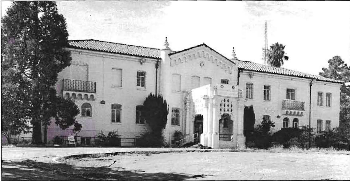
Building 515: Hospital (1934). Front elevation. The base hospital is a 3-story, concrete and stucco building designed under the direction of Captain Nurse. Laboratories and an X-ray room occupied the ground floor. The second floor contained offices, and the third floor housed operating rooms.
