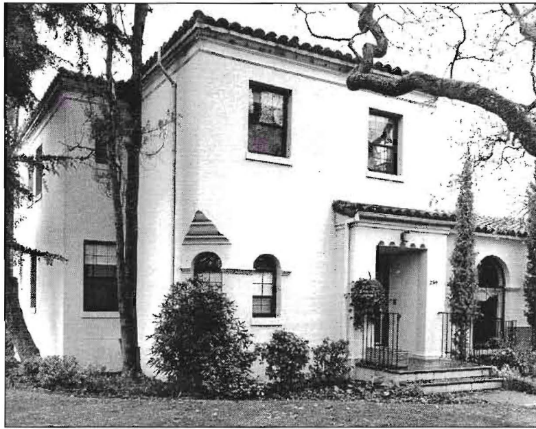
Building 299: Base Commander's Quarters (1934). Of the permanent housing units designed by Captain Nurse, the base commander's house was the largest and only one of its type at Hamilton. Architecturally, it is an H-shaped building with a hipped, Mission tile roof. It is two stories high on the north side and one story in height on the remaining sides. The house has five bedrooms, two bathrooms, a dining room, kitchen, card room, maid's quarters, basement, and a double garage.
