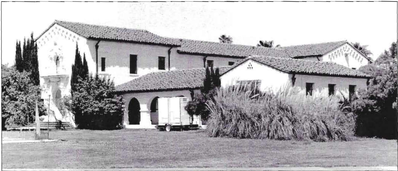
Building 500: Base Headquarters (1934). Front elevation. Designed in the Spanish Eclectic architectural style by Hamilton's Constructing Quartermaster Office under the supervision of Captain H. B. Nurse. This T-shaped building is constructed of concrete and features white stucco walls, Mission tile roofs, a Spanish Churrigueresque portal, decorative tilework, and arcaded walkways. The base headquarters was one of the first buildings completed on the base. It served as the group headquarters from its completion in 1934 until the Air Force vacated the base in 1975.
