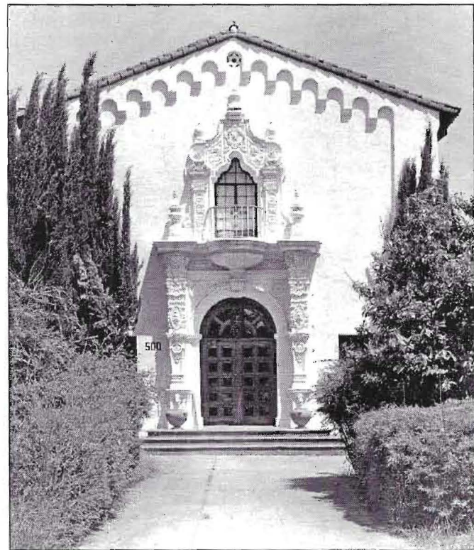
Building 500. Front facade of Base Headquarters Building with Churrigueresque entry.
