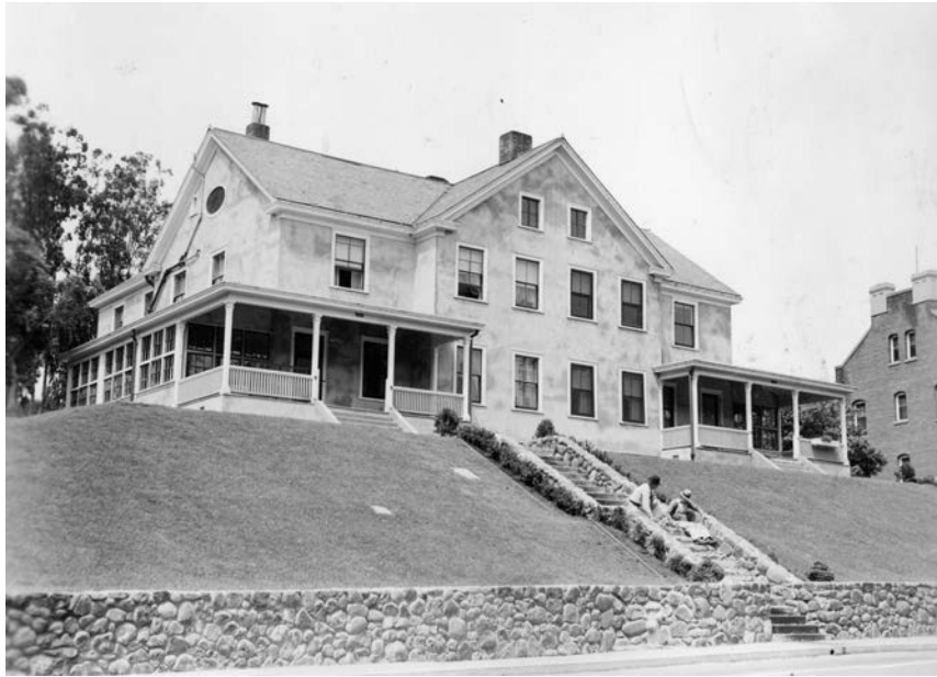
Quarters 26 A&B, Fort Winfield Scott, Schonher's quarters. NARA, RG 77, Entry 393, Box 237
