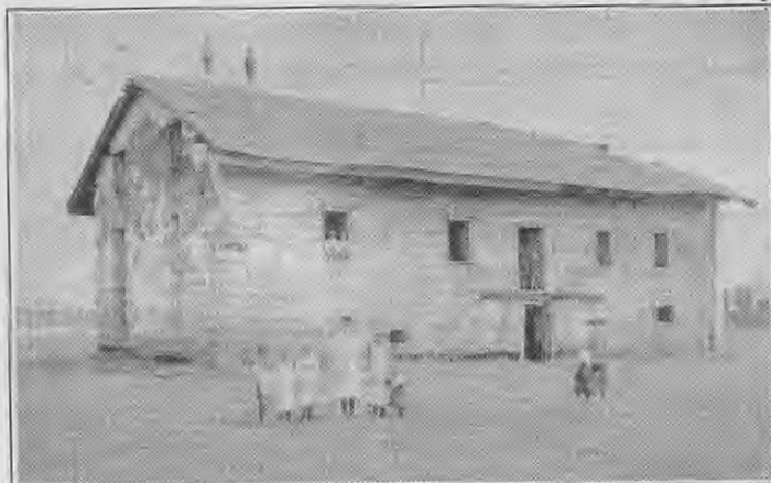
MAIN HOUSE IN DETERIORATED CONDITION
