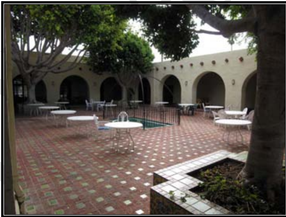
Plate 9. F-Troop Building, interior courtyard (Photo by RCGA, Inc., 2007)
