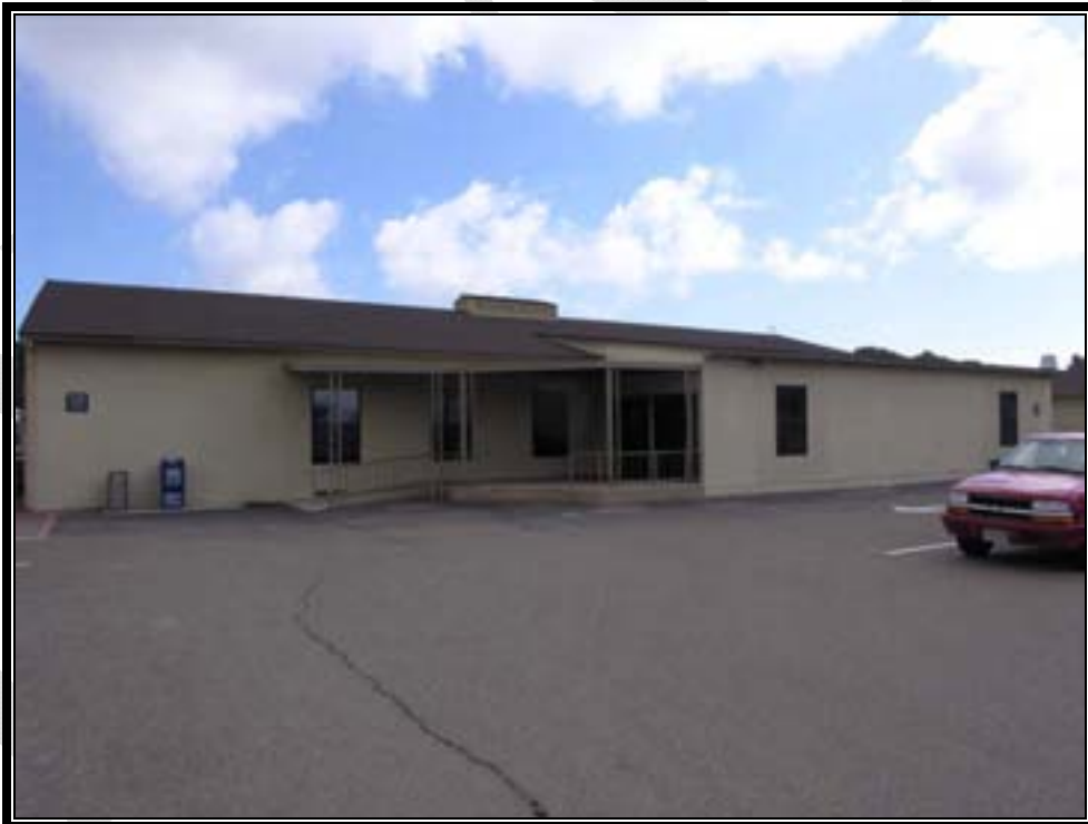
Plate 30. Building 864, central lounge exterior (Photo by RCGA, Inc., 2007)
