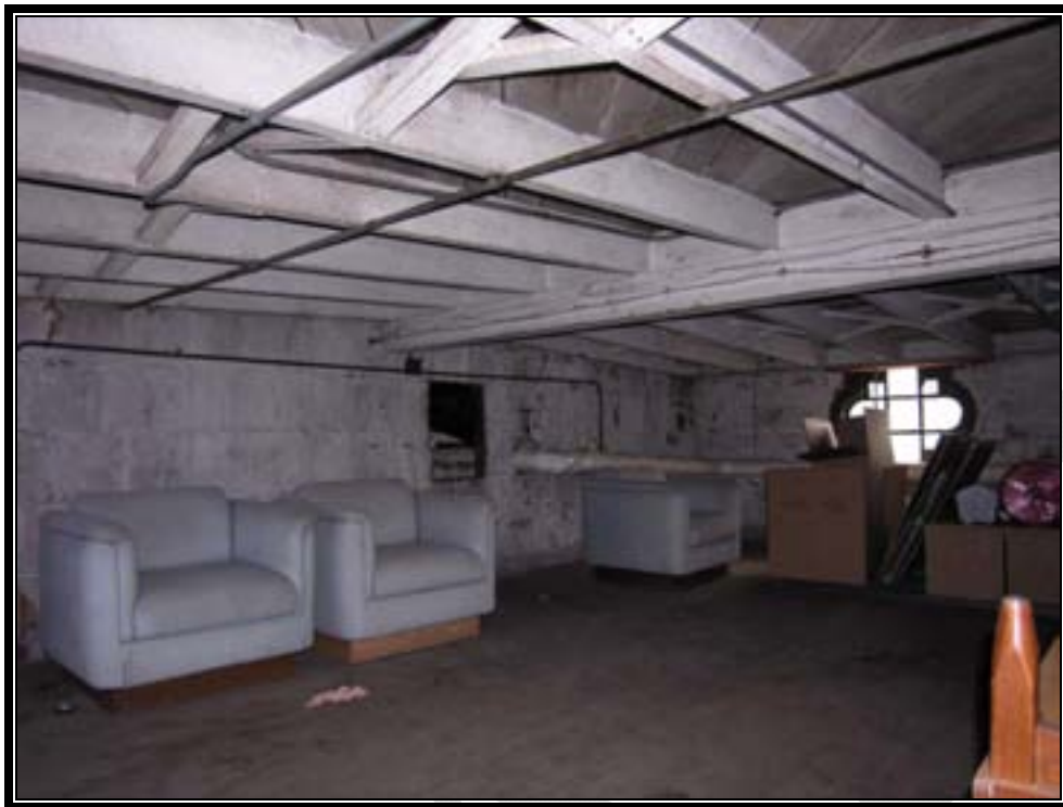
Plate 11. F-Troop attic (Photo by RCGA, Inc., 2007)
