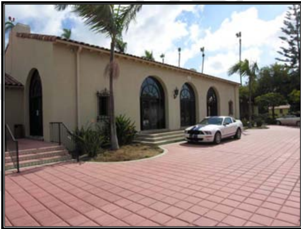
Plate 16. Building I, entry detail (Photo by RCGA, Inc., 2007)
