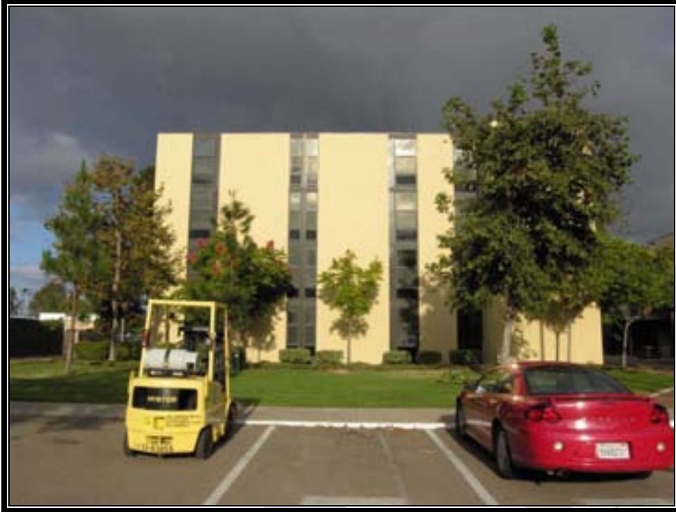
Plate 40. Building 776, east elevation view west (Photo by RCGA, Inc., 2007)
