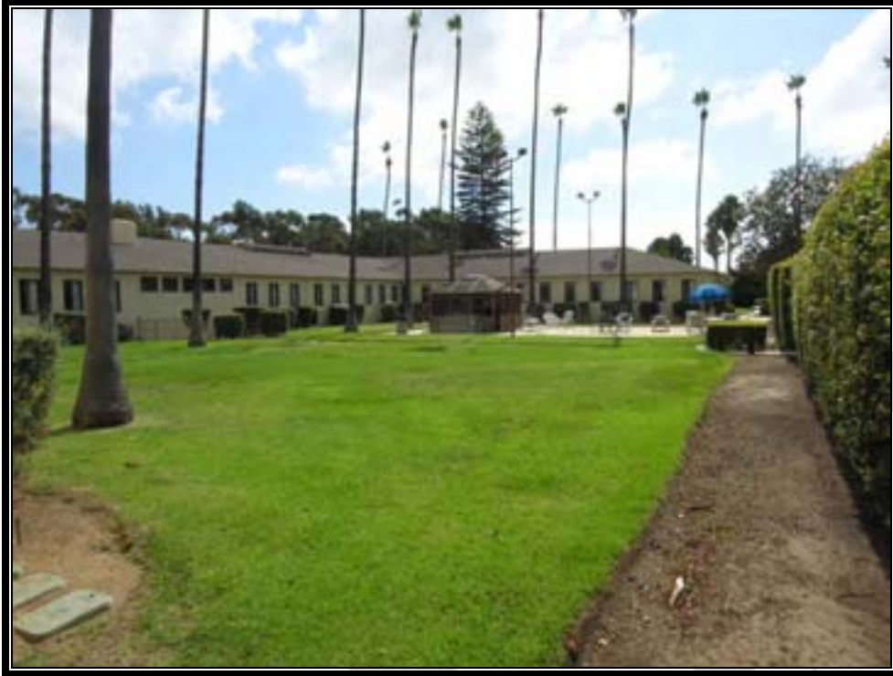
Plate 19. Building I, courtyard of extension (Photo by RCGA, Inc., 2007)
