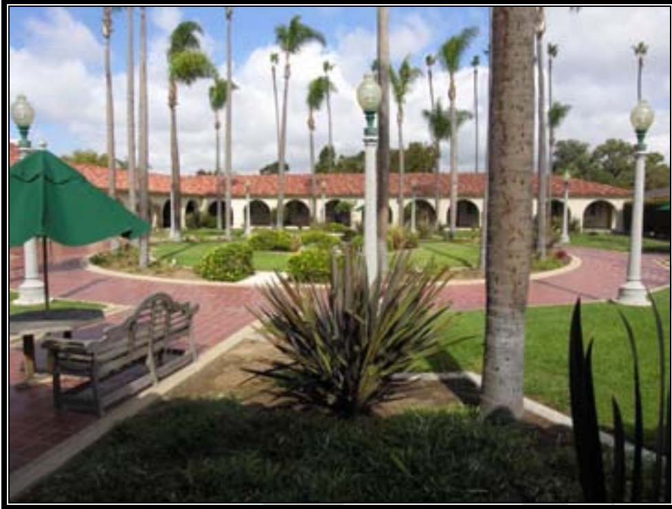
Plate 17. Building I, overview of courtyard (Photo by RCGA, Inc., 2007)
