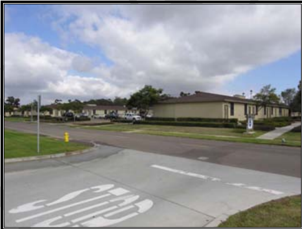
Plate 28. Building 864, overview looking northeast (Photo by RCGA, Inc., 2007)
