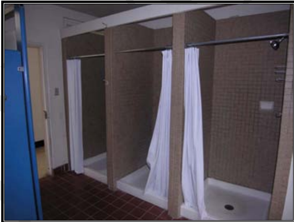
Plate 14. F-Troop Building, communal shower/restroom (Photo by RCGA, Inc., 2007)
