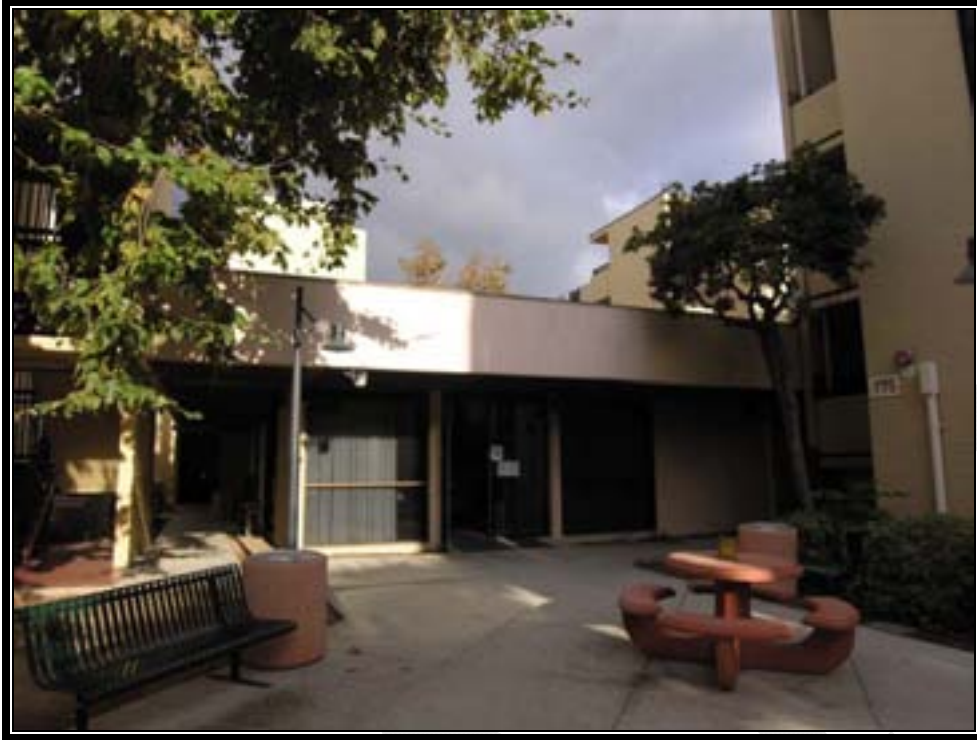
Plate 42. Building 773, central lounge, exterior (Photo by RCGA, Inc., 2007)
