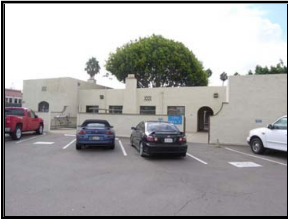
Plate 8. F-Troop Building north elevation (Photo by RCGA, Inc., 2007)
