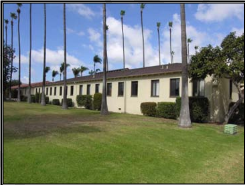
Plate 20. Building I extension, south elevation (Photo by RCGA, Inc., 2007)
