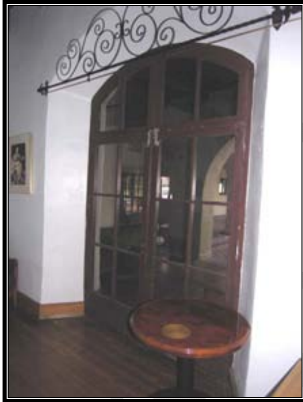
Plate 15. F-Troop Building, entry to CPO Club (Photo by RCGA, Inc., 2007)
