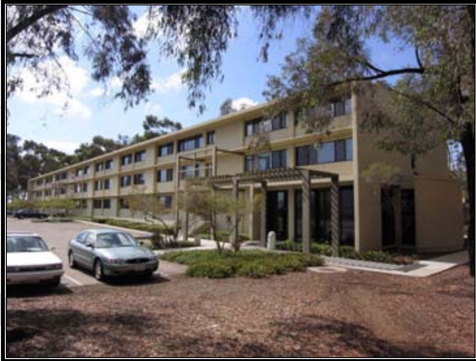
Plate 37. Building 572, east elevation looking southwest
