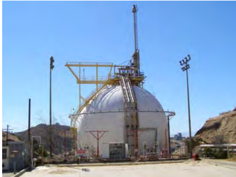
Photo 4.43. Vessel V100, LH2 tank, camera facing southwest. (Source: Archaeological Consultants, Inc., 2007.)
