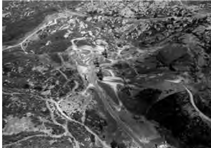
Photo 3.14. Alfa site at AFP 57 (NASA Area II), 3 June 1958. Pre-test building, Alfa I, II, and III test stands, underground blockhouse facing the spillway ravine (foreground right), pill box (center right), 24-inch aboveground pipeline to water storage tanks (background to upper right corner), and fuel infrastructure.
