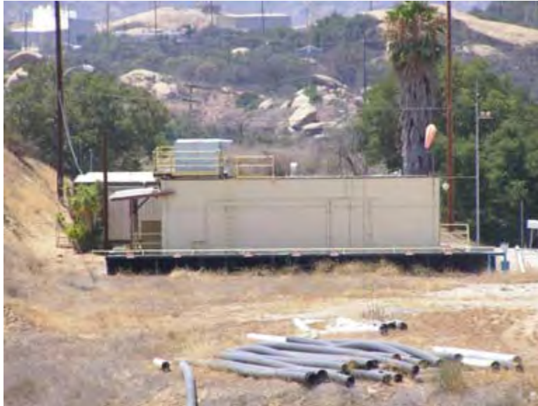
Photo 4.16. Alfa Control House, east elevation, which faces test stands. (Source: Archaeological Consultants, Inc., 2007.)
