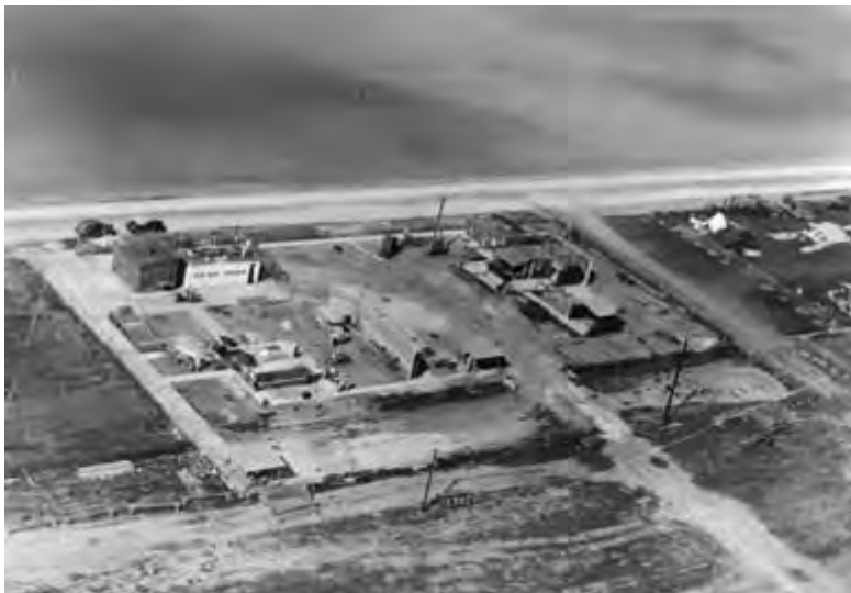
Photo 3.2. North American Aviation's makeshift rocket engine test site, neighboring its plant at the Los Angeles Airport, 1947.
