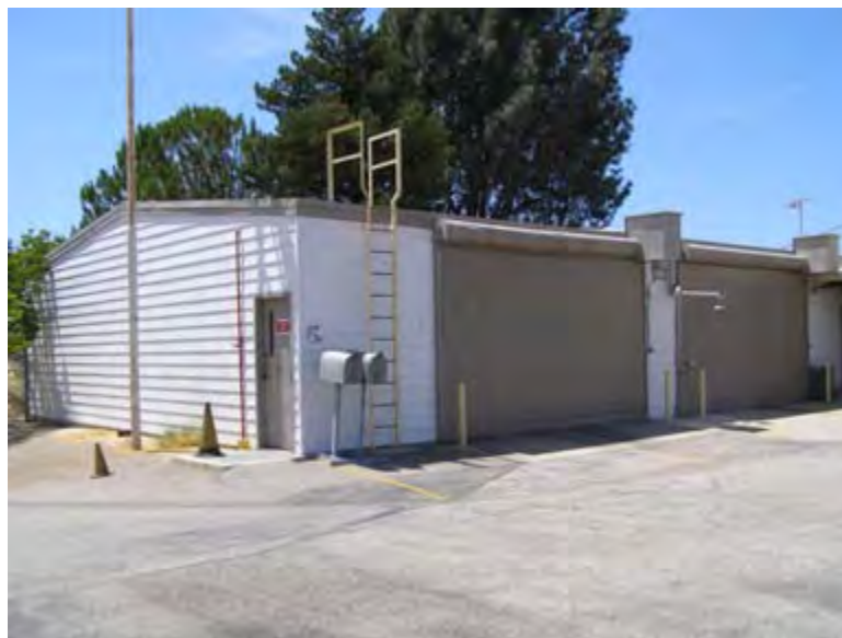
Photo 4.5. Alfa Pre-Test Building, camera facing north. (Source: Archaeological Consultants, Inc., 2007.)
