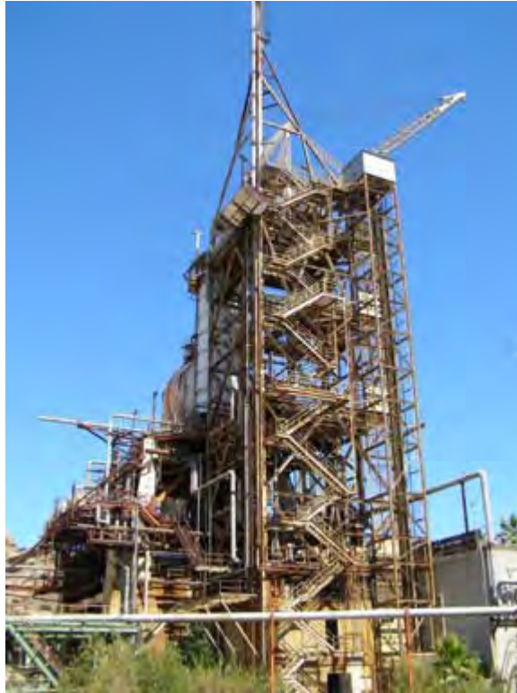
Photo 4.51. Coca I Test Stand, west elevation. (Source: Archaeological Consultants, Inc., 2007.)
