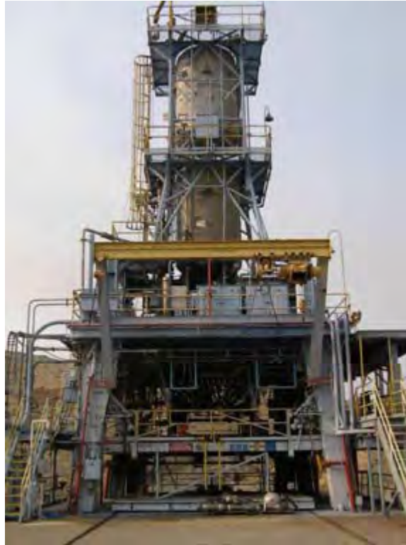
Photo 4.6. Alfa I Test Stand, north elevation. (Source: Archaeological Consultants, Inc., 2007.)
