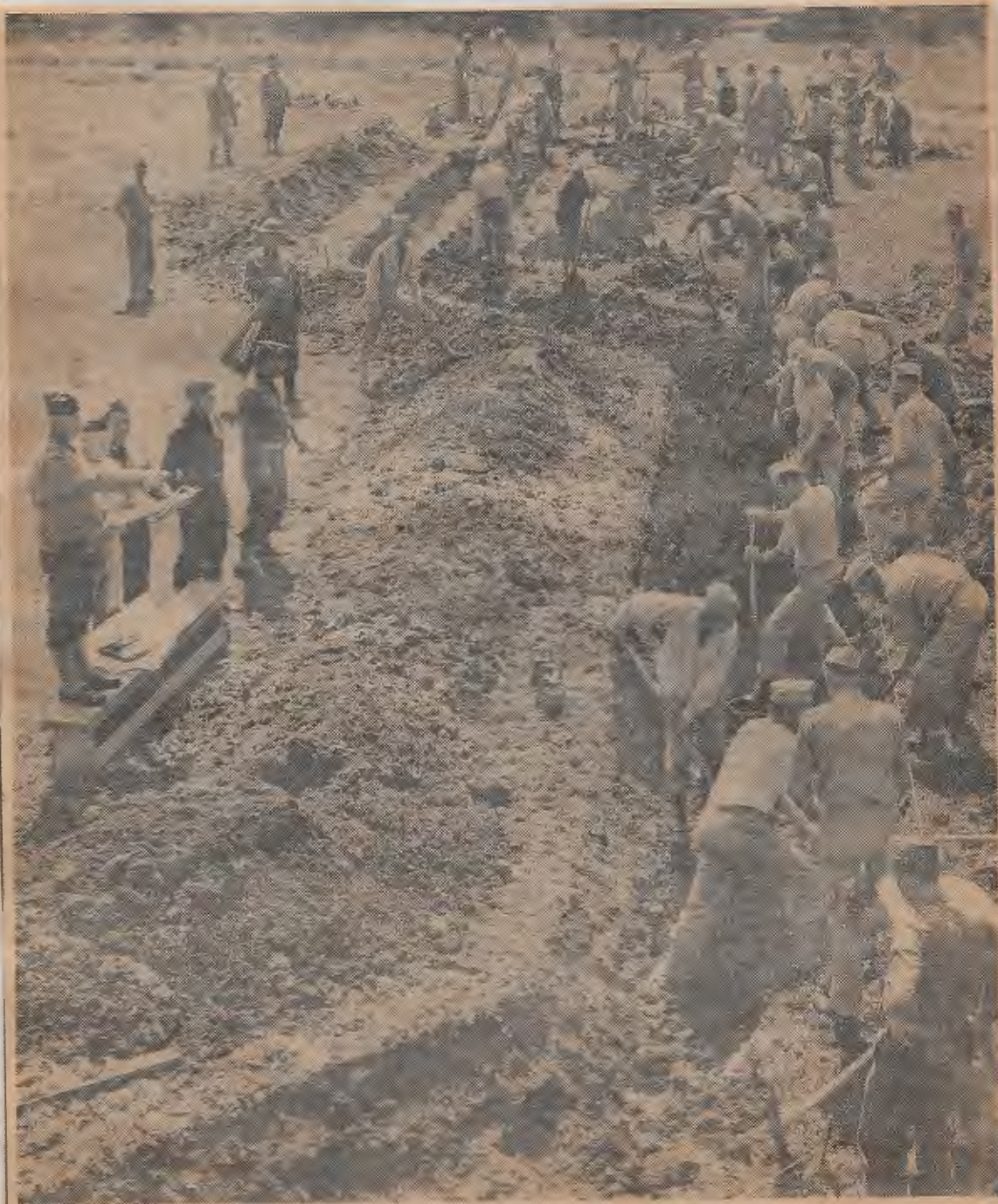
DIGGING IN —Maj. Henry L. Hart, extreme left, with map, directs men of 1st Engineers Regiment, California State Guard, in demonstration of trench digging yesterday.
