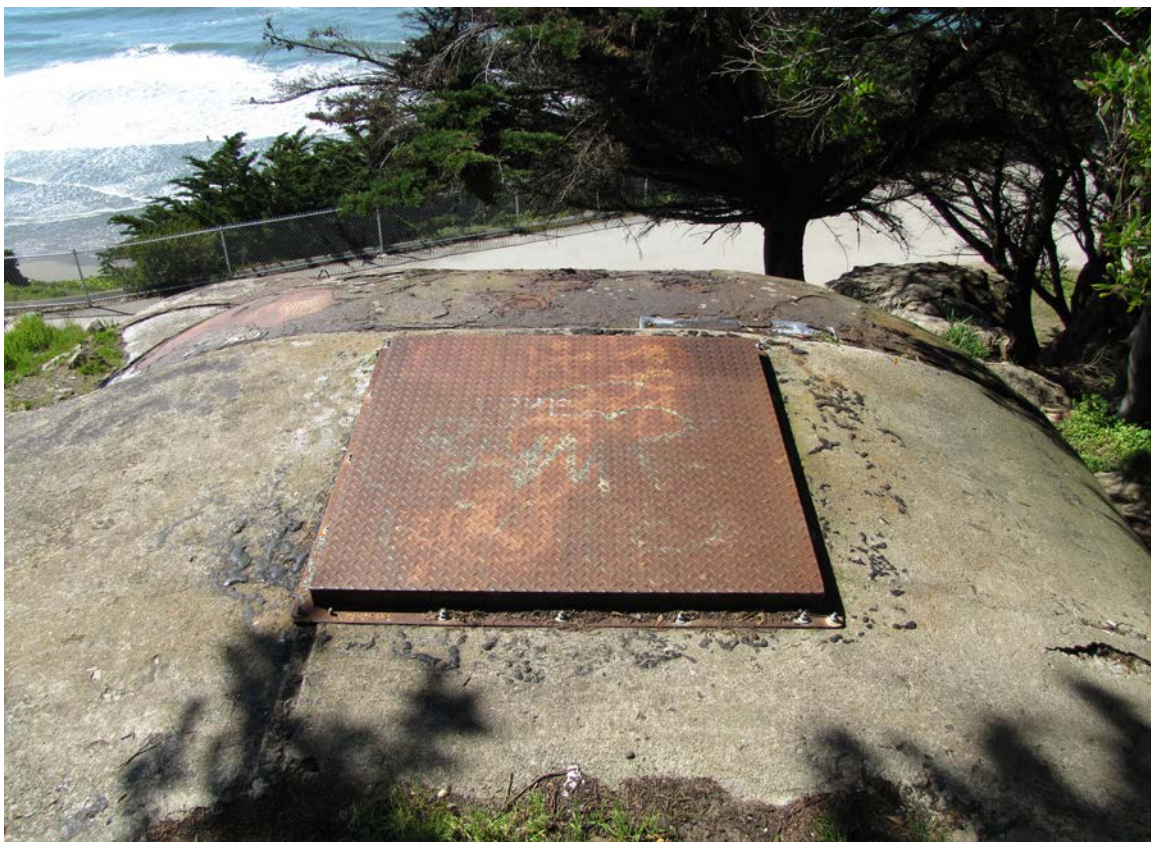
Figure 11. New steel cover for B 2 S 2 BCN 129 manhole. Photograph by author, March 2017.
