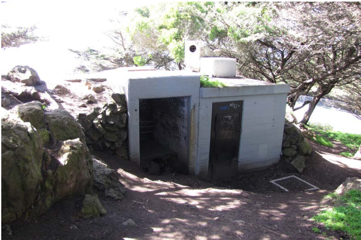
Figure 7. Left to right - entrance way to the double base end station and steel door to the power house.
