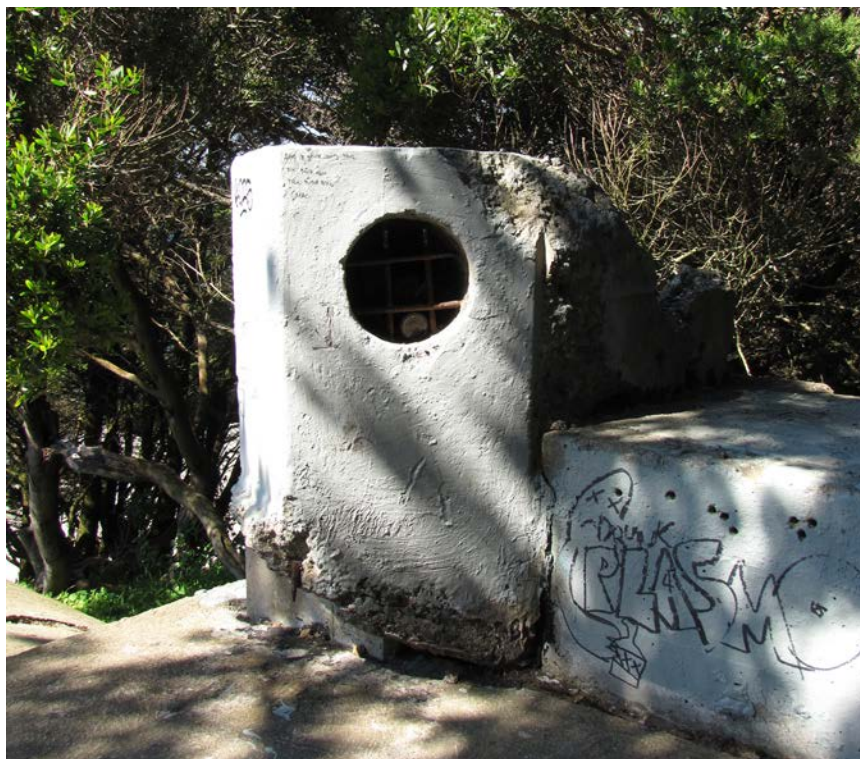
Figure 9. Concrete vent for B 2 S 2 BCN 129. Photograph by author. March 2017.
