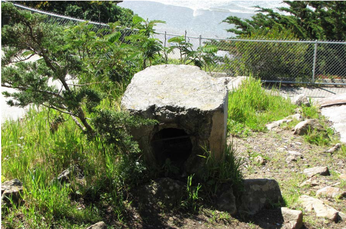
Figure 10. Concrete vent for M 3 Mines II base end station. Photograph by author, March 2017.
