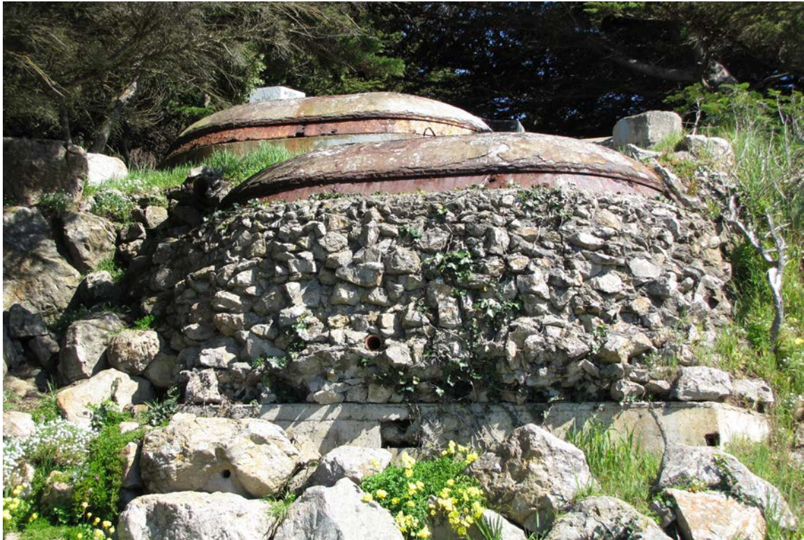
Figure 6. M 3 Mines II with local rock façade. The base end station for B 2 S 2 BCN 129 is directly above.
