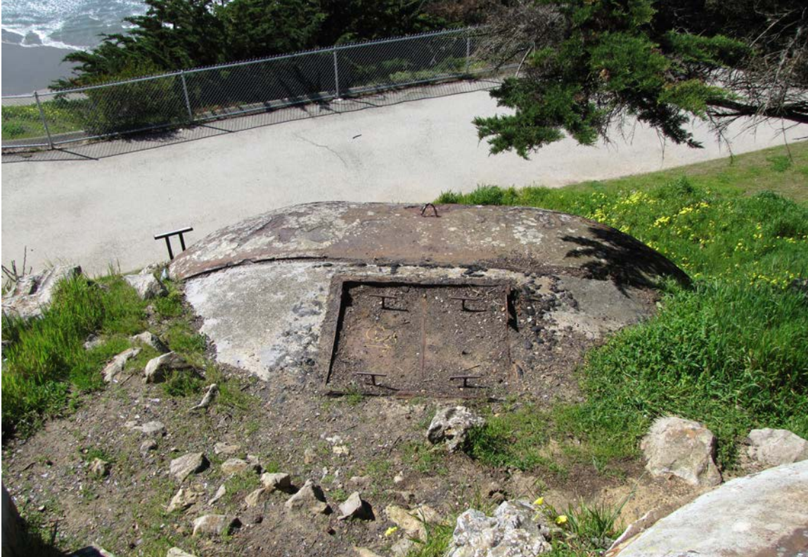
Figure 12. Sealed manhole for the M 3 Mines II base end station. Photograph by author, March 2017.
