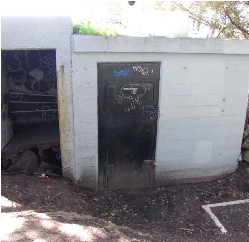
Figure 8. Current steel door to the Sutro Heights powerhouse. Note the sealed vent for the powerhouse. Photograph by author. March 2017.
