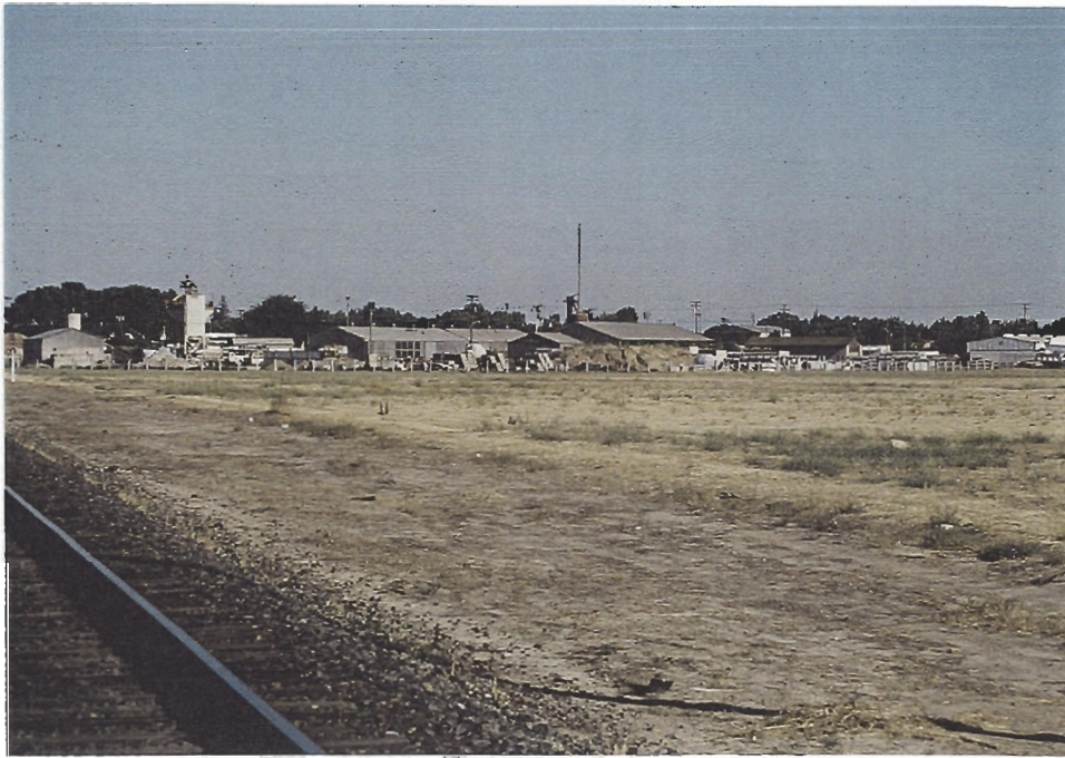
PHOTO # 1 NORTHERN PORTION OF THE SITE - CONCRETE PIPE MANUFACTURER
