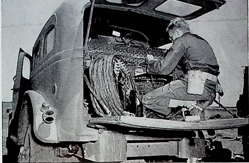
SIGNAL COMPANY TACKLES PROBLEM OF WIRE LAYING
