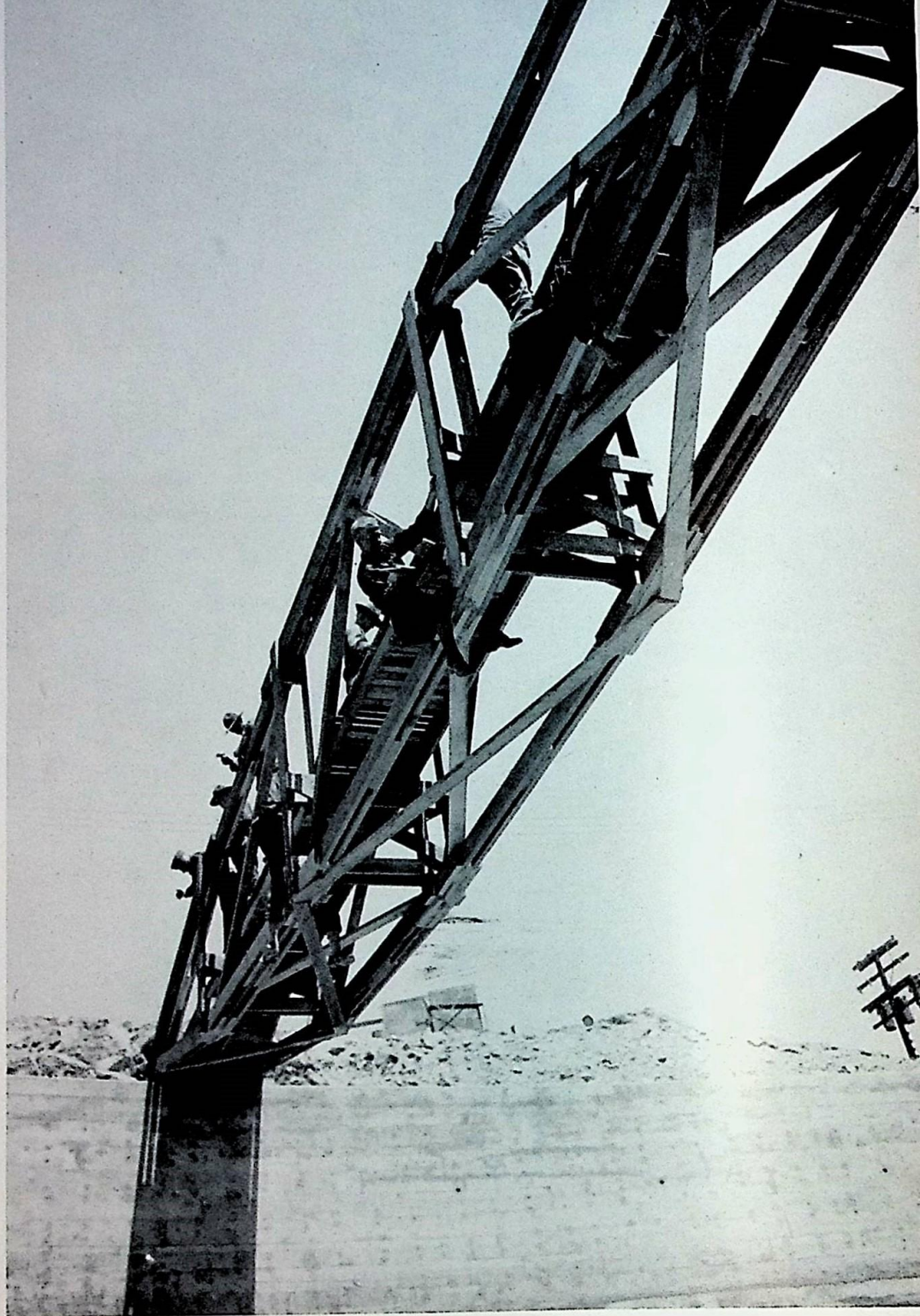
115th Engineers build a Pauli-Truss footbridge spanning reservoir spillway.
