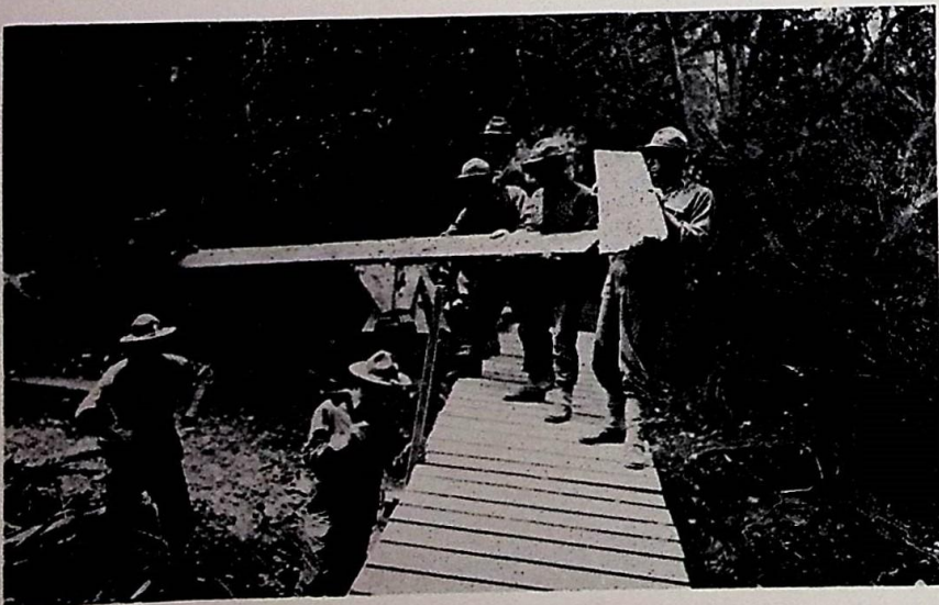
CREW BUILDS BRIDGE ACROSS CREEK
