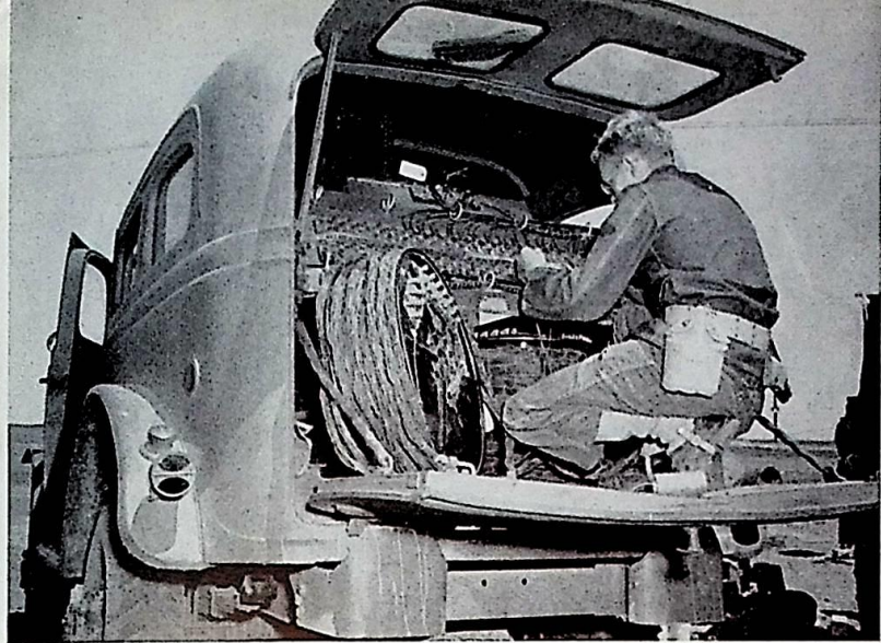
SIGNAL COMPANY TACKLES PROBLEM OF WIRE LAYING
