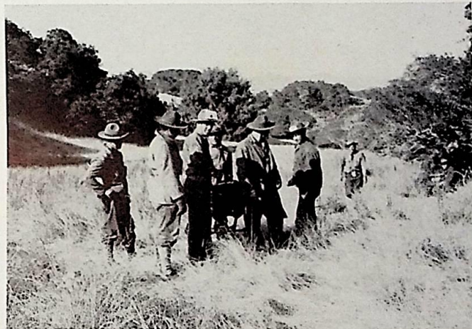
Left, telephone wire is laid by a crew in the field.
