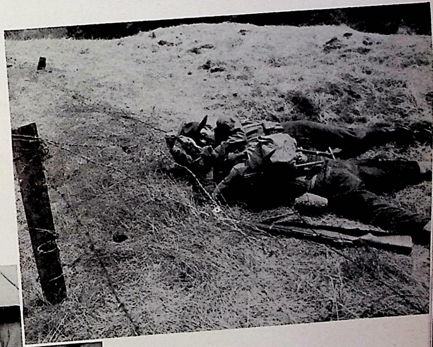
Top: Sighting a trench mortar. Top Right: Men in a communication trench. Bottom: Planning action. Right: Wire cutting detail.
