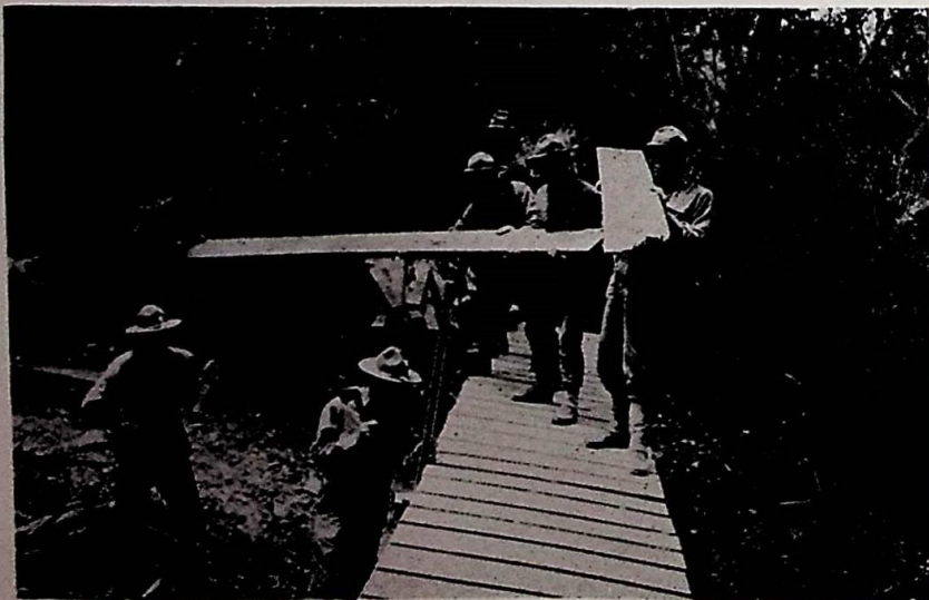
CREW BUILDS BRIDGE ACROSS CREEK
