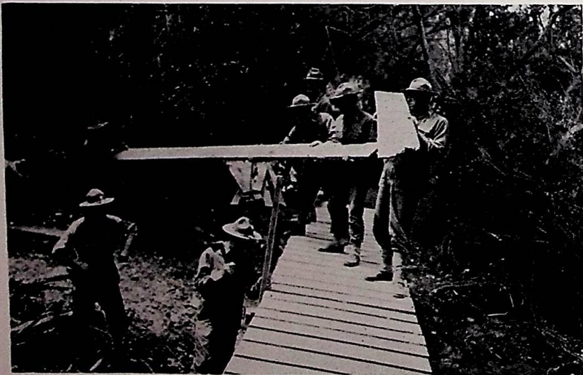
CREW BUILDS BRIDGE ACROSS CREEK
