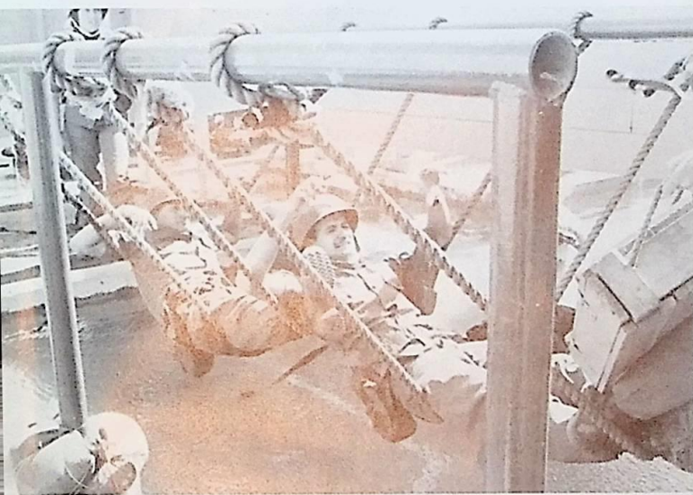
The Cadet bridge planks are in place
