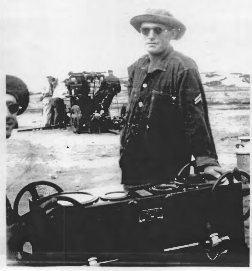
WE LATER RECEIVED 37 MM AND LATER 40 MM CANNONS THAT HAD ELECTRIC DIRECTORS AND DRIVEN BY OIL GEAR MOTORS POWERED BY ELECTRIC MOTORS (EACH GUN HAD A 3,000 WATT GENERATOR).
