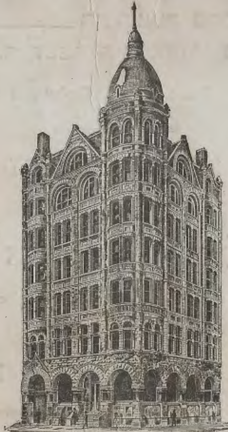
COMPANY'S BUILDING N. E. cor. Sacramento and Montgomery Sts.
