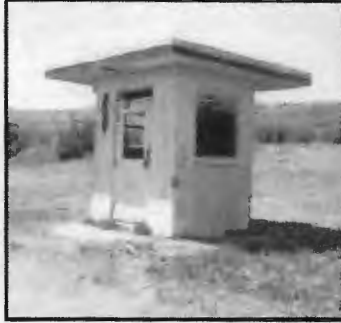
Access Area Guard Shack
