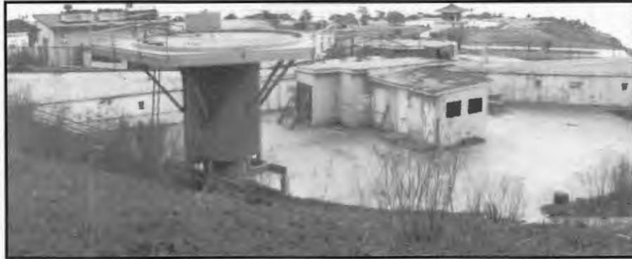
Integrated Fire Control (IFC) Area – Upper Reservation, Fort MacArthur
